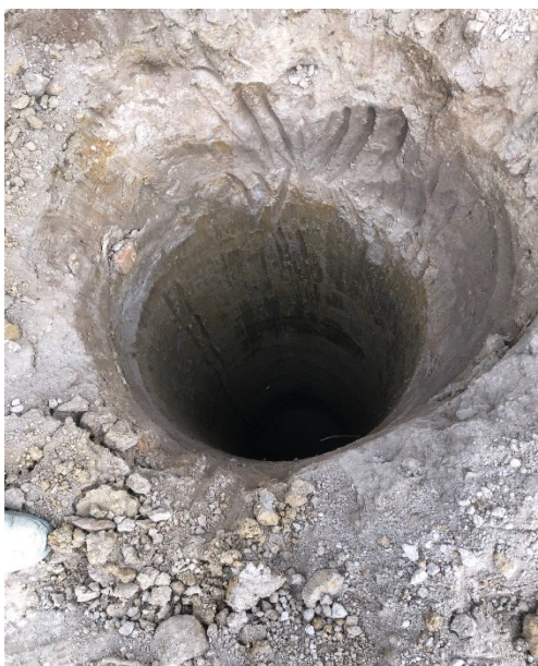
6 Metre Deep Pier Drilling
