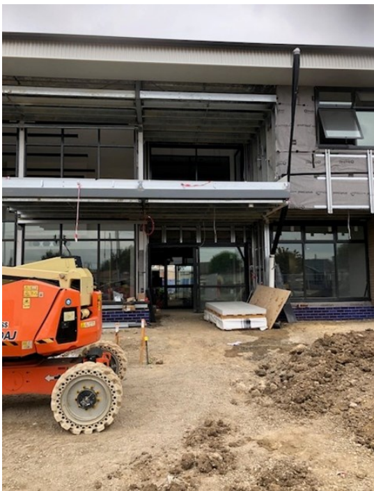
Construction of the front entrance of the Junior/Senior Campus
